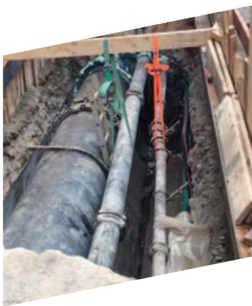
Pipes before removal
