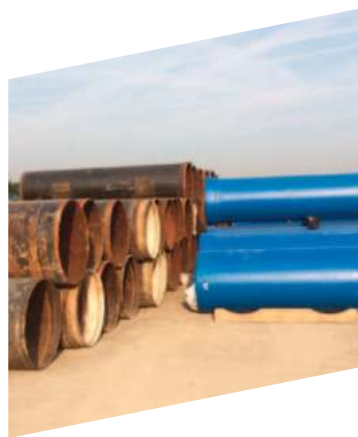
Storage of old and new pipes
