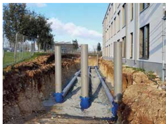
ELIXAIR® Earth-to-air heat exchanger
